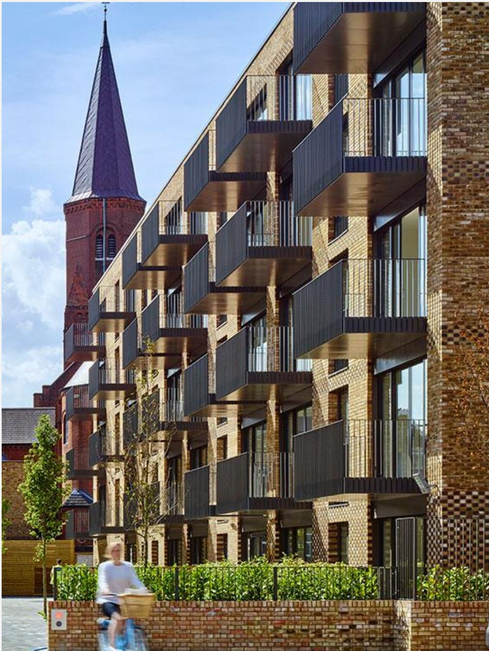
This is one of the first UK residential structures built out of cross-laminated timber (CLT). This durable structural material has the potential to save on energy costs due to its compact wood layers allowing only half the air leakage of concrete, which reduces the amount of energy needed to heat the building by 40 percent.
